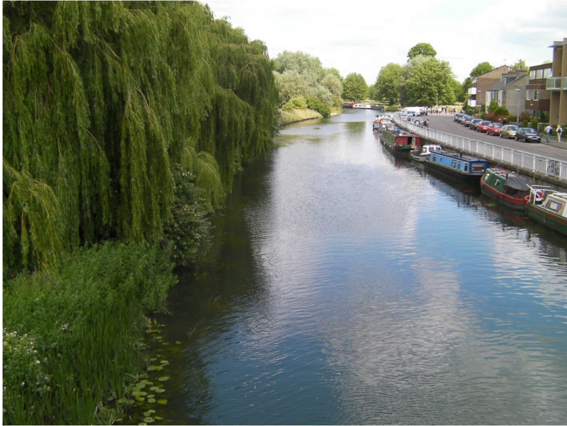
View of overhanging trees and reeds downstream from the new bridge.
