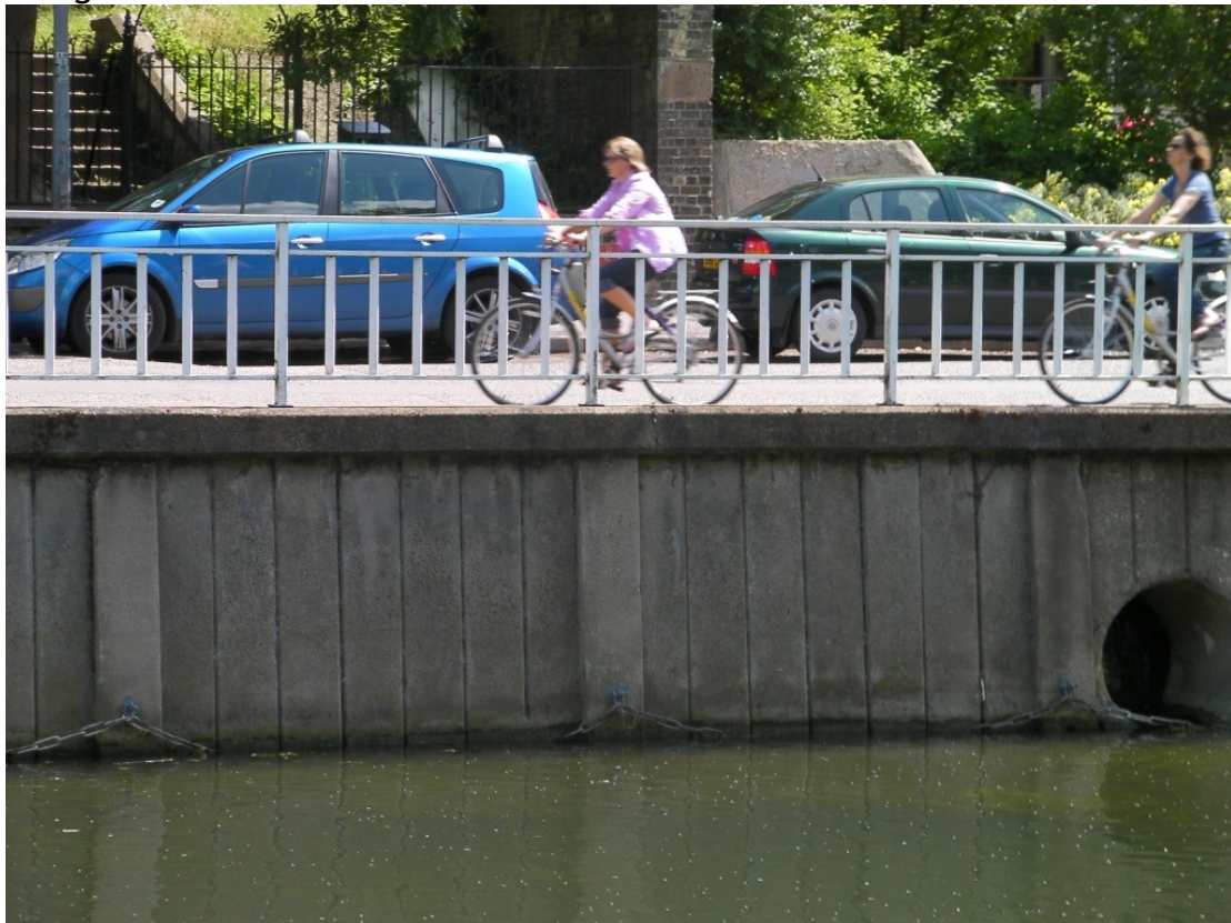
Grab chains and the retaining wall.
